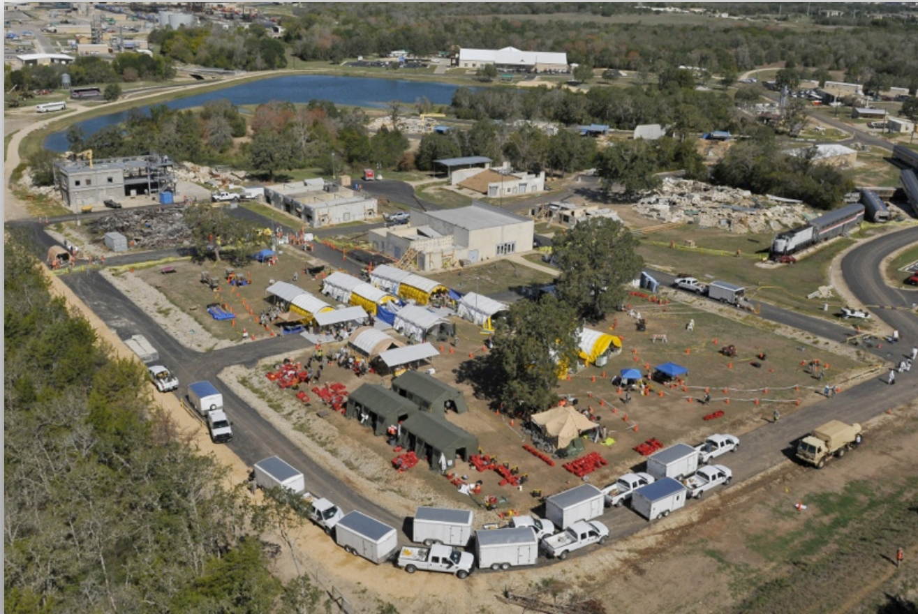
Disaster City, College Station, TX
